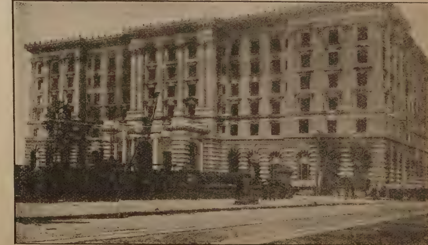
Partially finished Fairmount Hotel at Summit of Nob Hill, Interior damaged by fire
